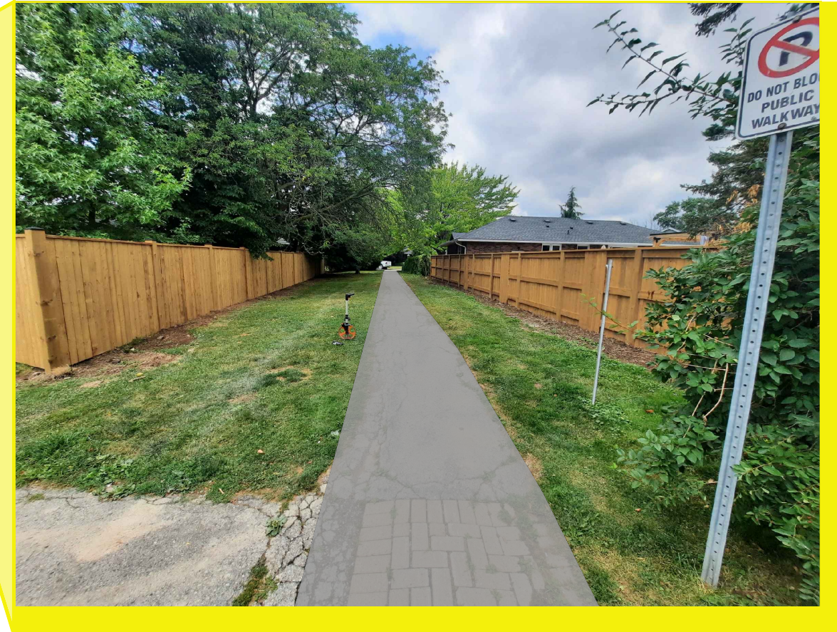
AFTER - CONCRETE WALKWAY LOOKING NORTH
